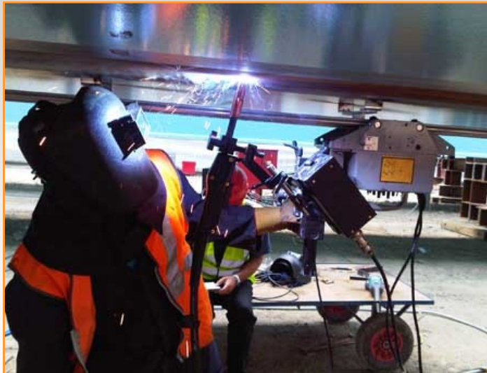
KAT Oscillation carriage combination welding overhead on Scottish bridge construction.
