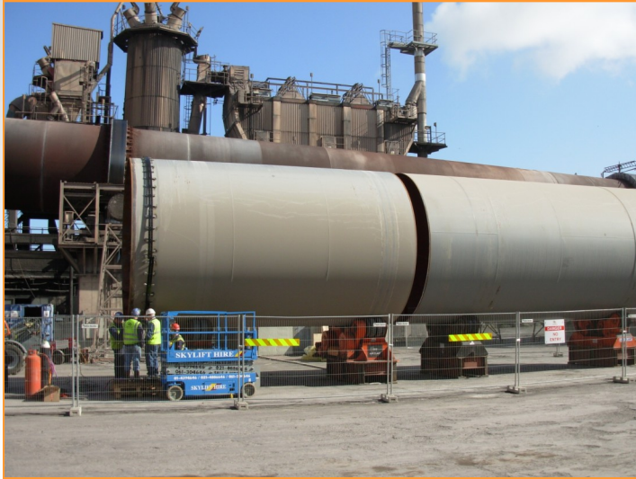
KAT® Automatic Travel Carriage with cutting package combination and flexible track mounted on a large kiln section.
