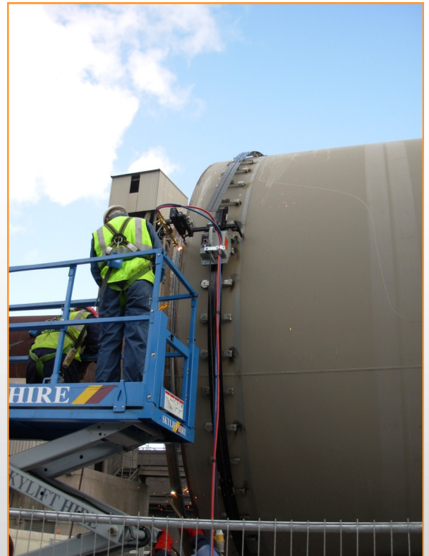
KAT® Automatic Travel Carriage cutting large kiln section in Ireland using the oxy-acetylene process.
