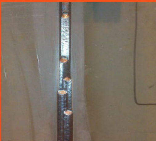
WELD - FRONT SIDE USING KAT® AUTOMATION
